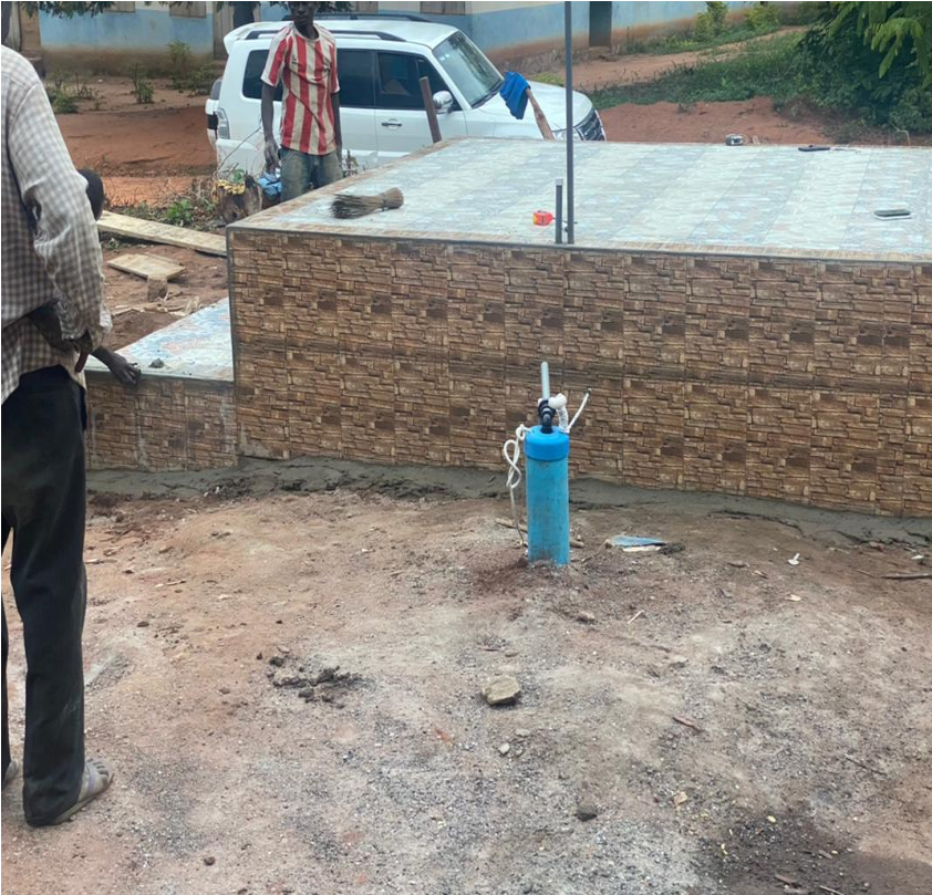
Construction of a Mechanized Borehole with Reservoir
